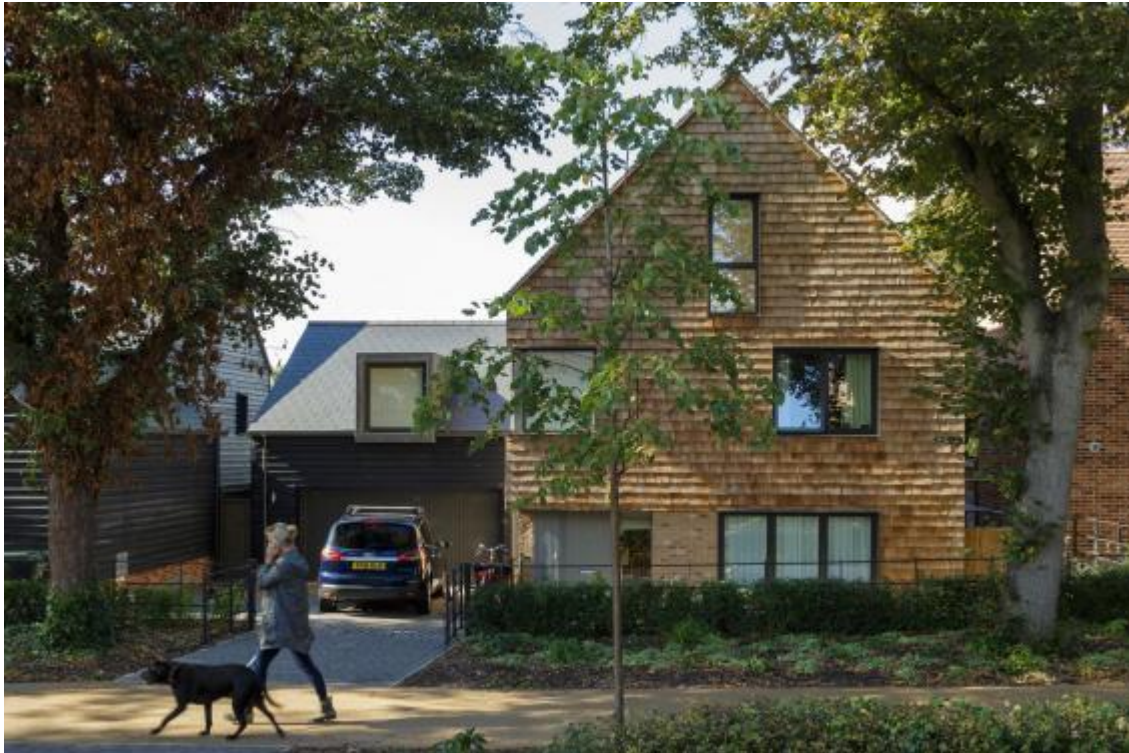
The Avenue in Essex is a new kind of housing estate (Tim Crocker)
